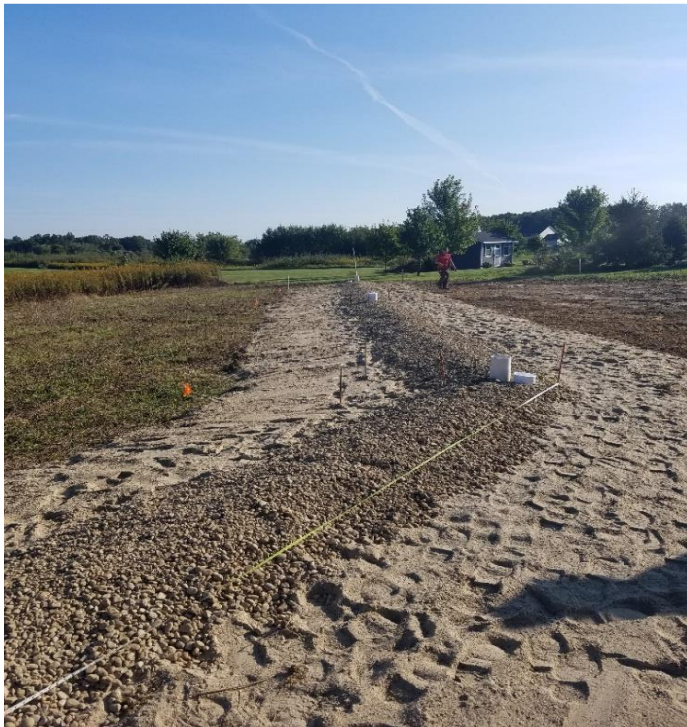
Inside of a Sand Mound System
